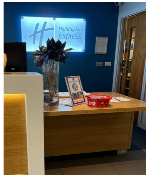
A lowered counter from Holiday Inn Express Walsall, UK
